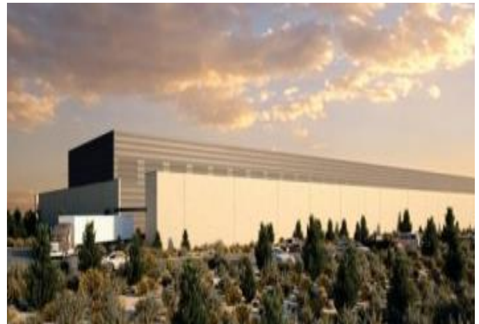
Figure 11: Facebook Data Center[29]
